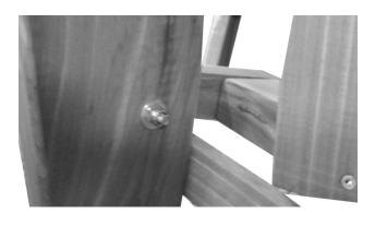
D. Secure Lag Bolt (A) with Washer (D) and Locking Nut (C) using 11mm or 7/16 socket.
